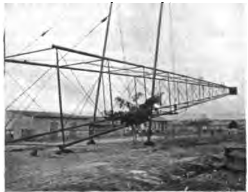
Aerial in course of erection.
